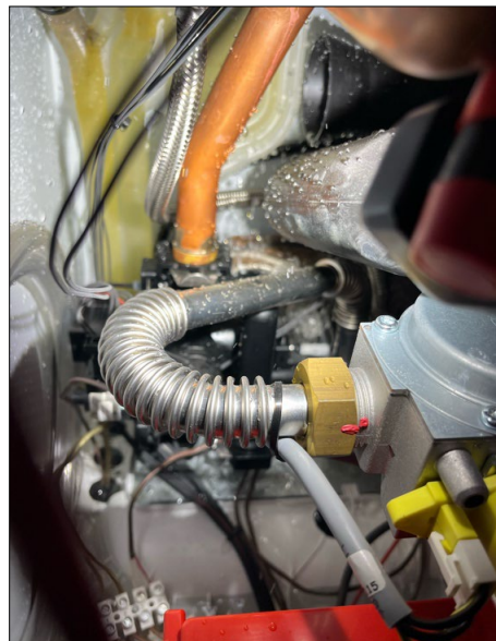
Leaking water in this boiler froze and damaged the heat exchanger.
