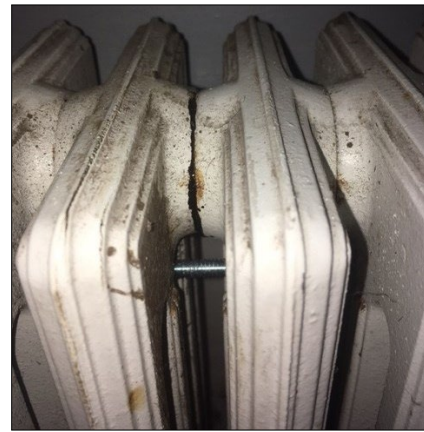
This radiator has cracked due to freeze damage and will need to be replaced.
